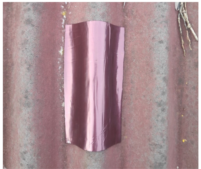
FIG 9 - ONDUBAND patch once applied
